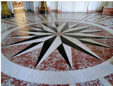
Marble floor in The Round Room in the Grand Trianon at Versailles Palace, made out of Carrara, black Belgium, and red Languedoc marble.
