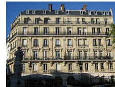
Haussmann building façade, place Saint Georges, Paris.
