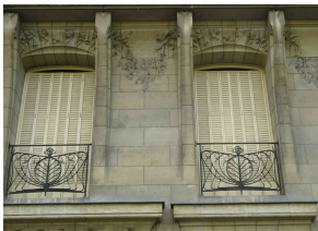
Detail of the first floor.
