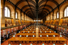
Metal covering of the reading hall of Sainte-Geneviève library by Labrousse, opened in 1851.
